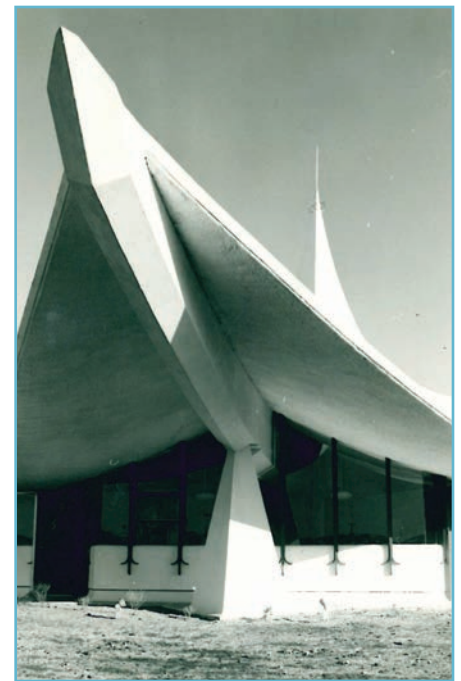
St. Stephen's Lutheran Church was named a historic location in August 2019.
