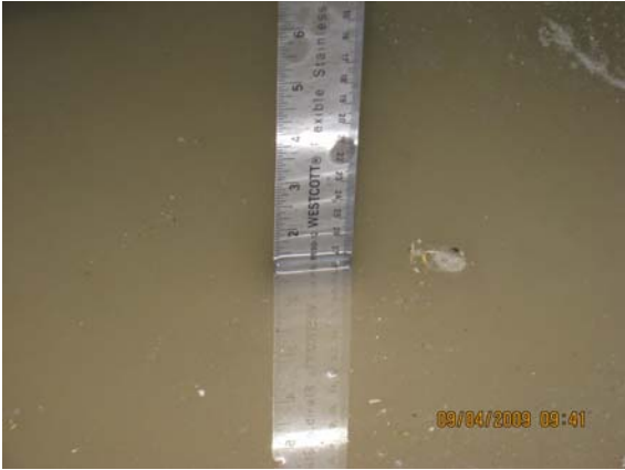
Pedestrian Underpass - West End Ponding
