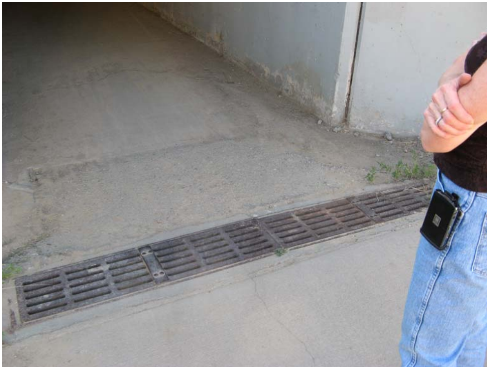
Pedestrian Underpass - East End Drain
