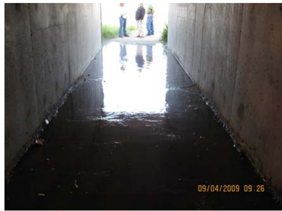
Pedestrian Underpass - West End Ponding
