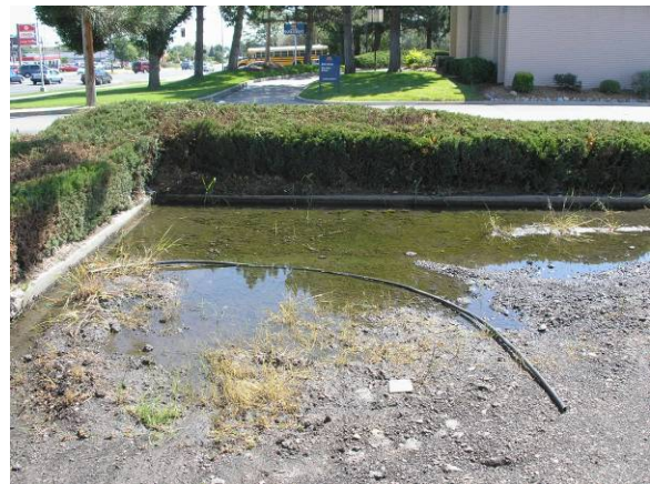
Makeshift Detention Pond
