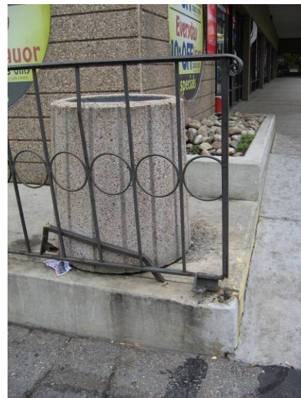
Broken Handrail
