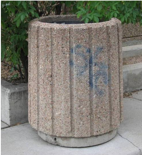
Graffiti on Trash Receptacle
