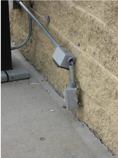
Exposed Wiring
