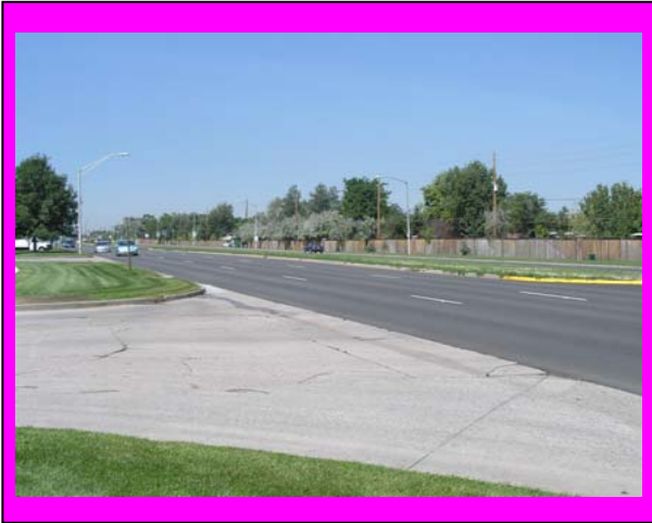
104 th from Zuni St. to Croke St. No Raised Median
