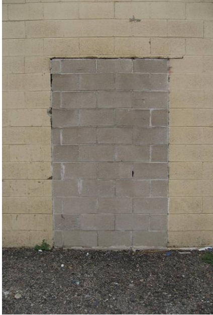
Doorway Permanently Sealed
