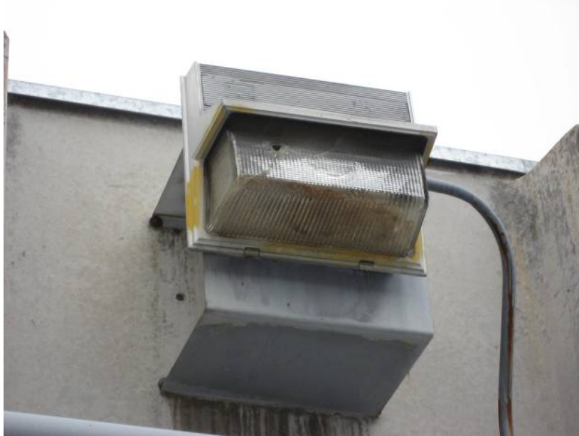
Exterior Light w/ Bullet Hole
