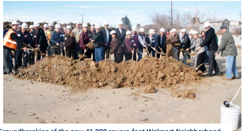
Groundbreaking of the new 41,000 square-foot Walmart Neighborhood Market grocery and pharmacy.
