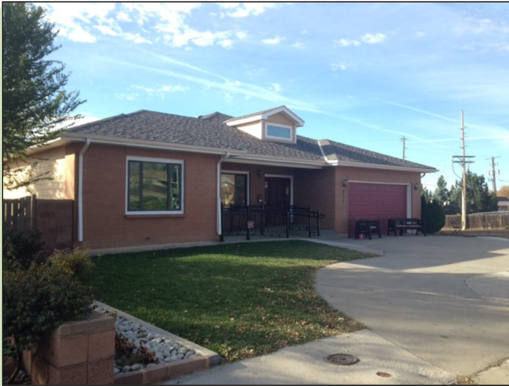
Front of existing assisted living home
