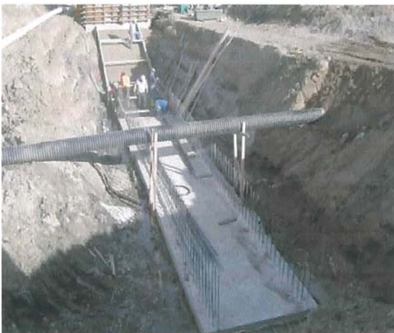
View east of center section of box culvert floor
