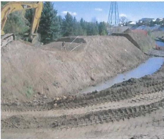
East embankment grading and fuse plug
