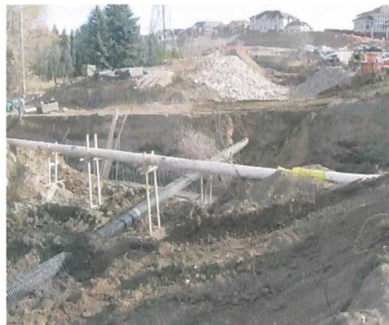
View southeast of pipe diversions over culvert trench
