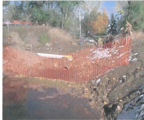
View east from existing inlet structure
