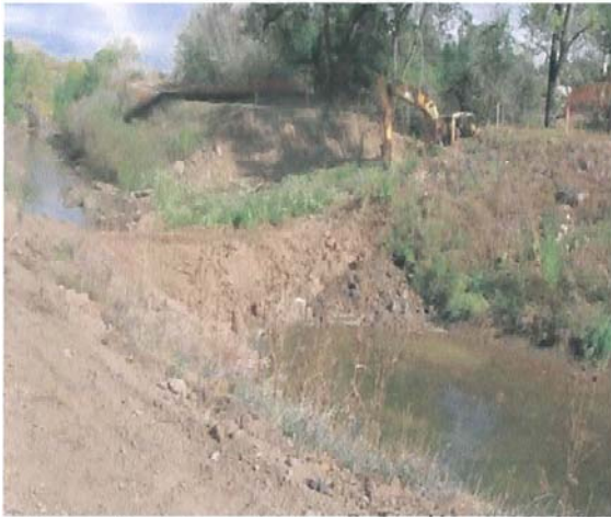
Excavation into east side embankment
