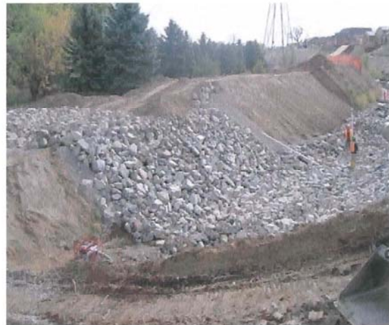
View southeast of riprap placement
