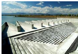
Labyrinth Spillway at Standley Lake
