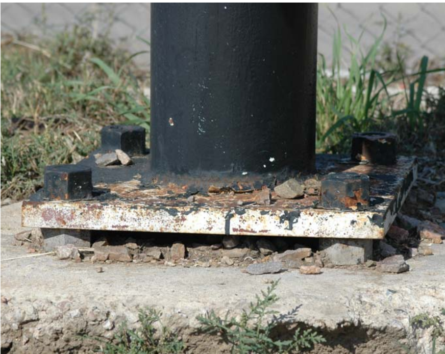
5.5.4. Base of sign.
