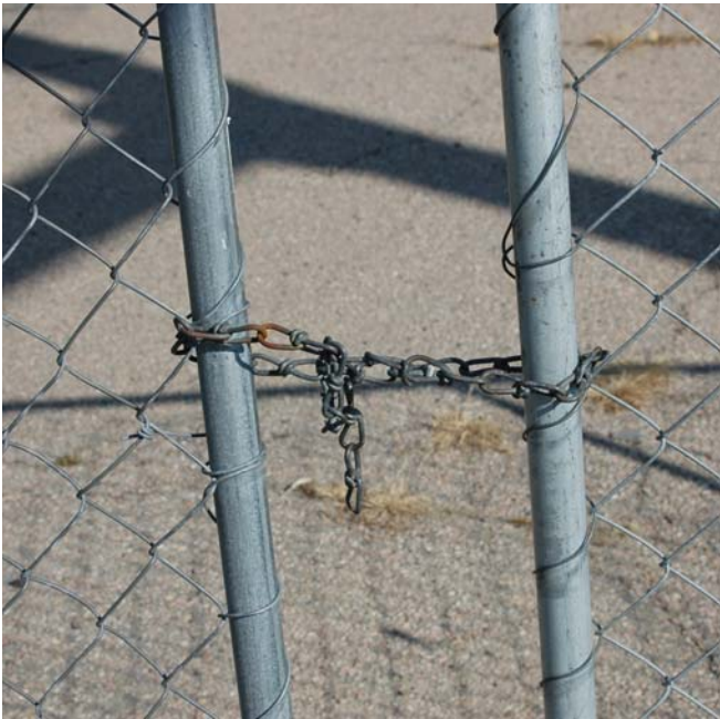
5.8.2. Site unsecured. No lock on gate.
