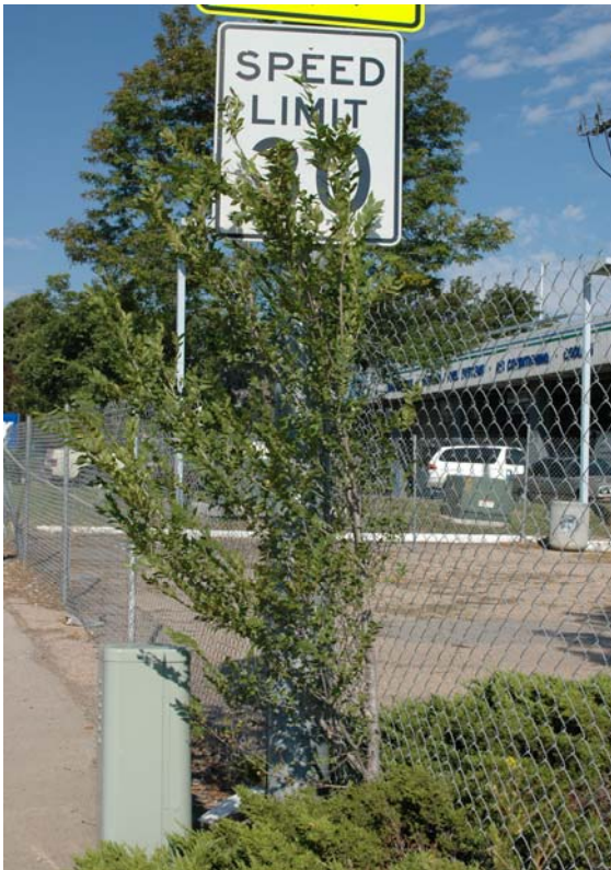
5.4.6. Tree obstructing traffic sign.
