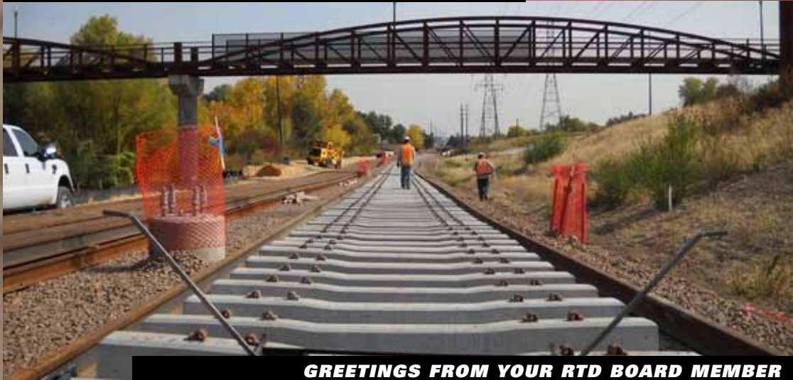
Crews installing light rail track on the West Corridor.
