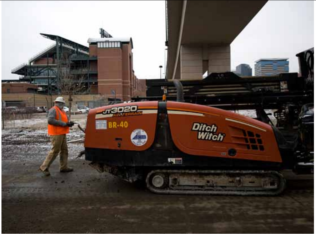
Construction worker starts the relocation of a major fiber optic cable for RTD's East commuter rail line to Denver International Airport.
