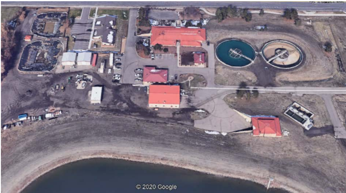
Figure 1-1: Northglenn WTP Existing Site Overview
