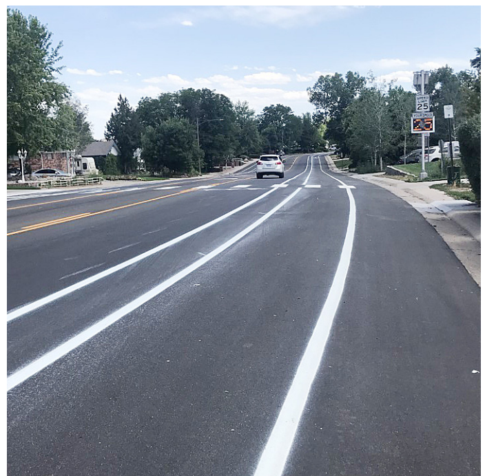
Through the Connect Northglenn Bicycle and Pedestrian Master Plan, pedestrian improvements, including bike lanes with buffers from vehicles, were added to Melody Drive.
