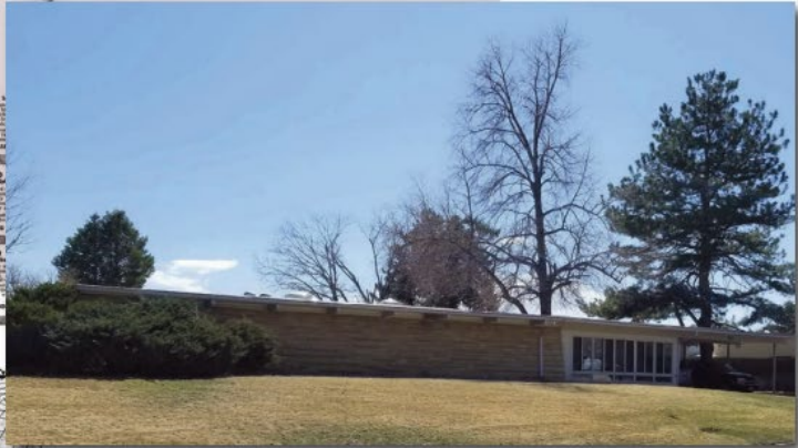
Parade of Homes advertising directed prospective buyers throughout metro-Denver to 840 W. 99th Avenue, a home that features a double carport, high-end stone siding, a flat roof with overhanging eaves and exposed rafter ends, and multiple patios. (Advertisement: Denver Post , 14 October 1956; Photo: Mary Therese Anstey)
