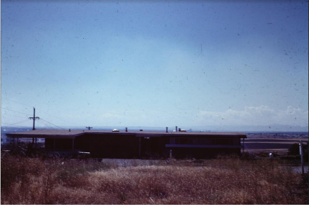
3 of 6: 880 W. 99 th Ave, exterior, date unknown.
