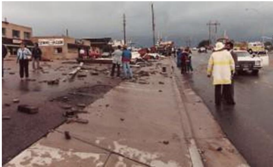
Figure 4-31 June 3, 1981, Tornado Damage Along Washington Street (Source: City of Thornton)
