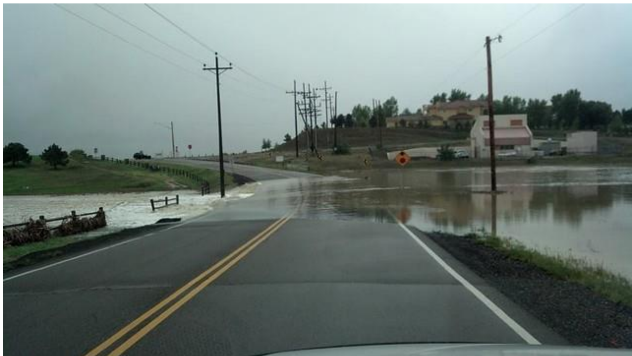
Figure 4-15 2013 Flooding in Thornton
