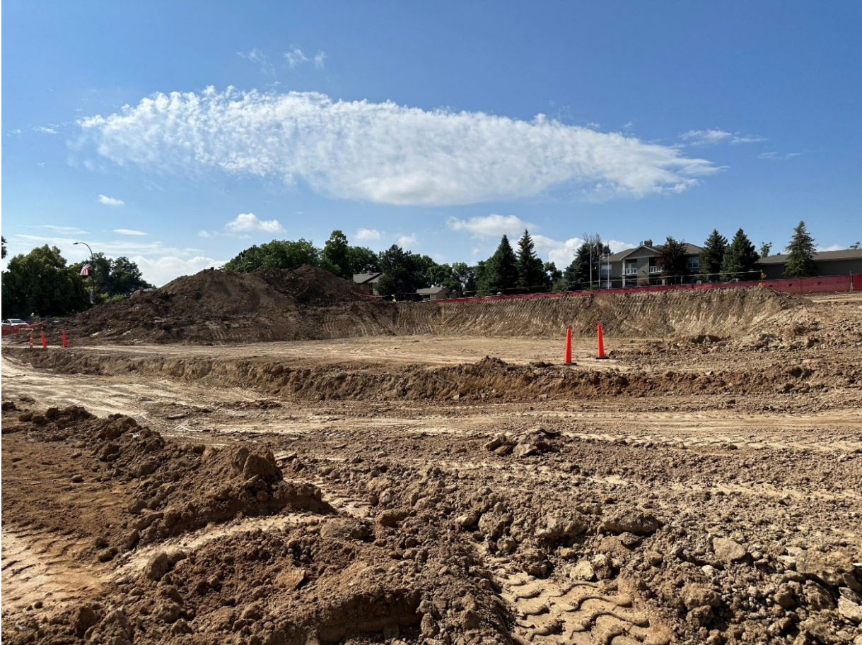
Photo 1 – Site Grading for First Level
