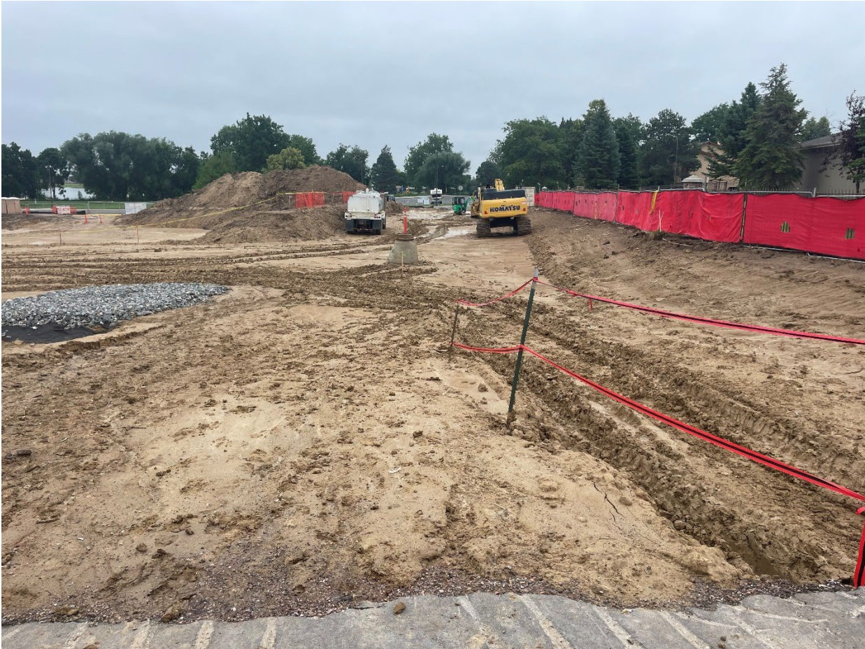
Photo 3 – South Access Drive Grading
