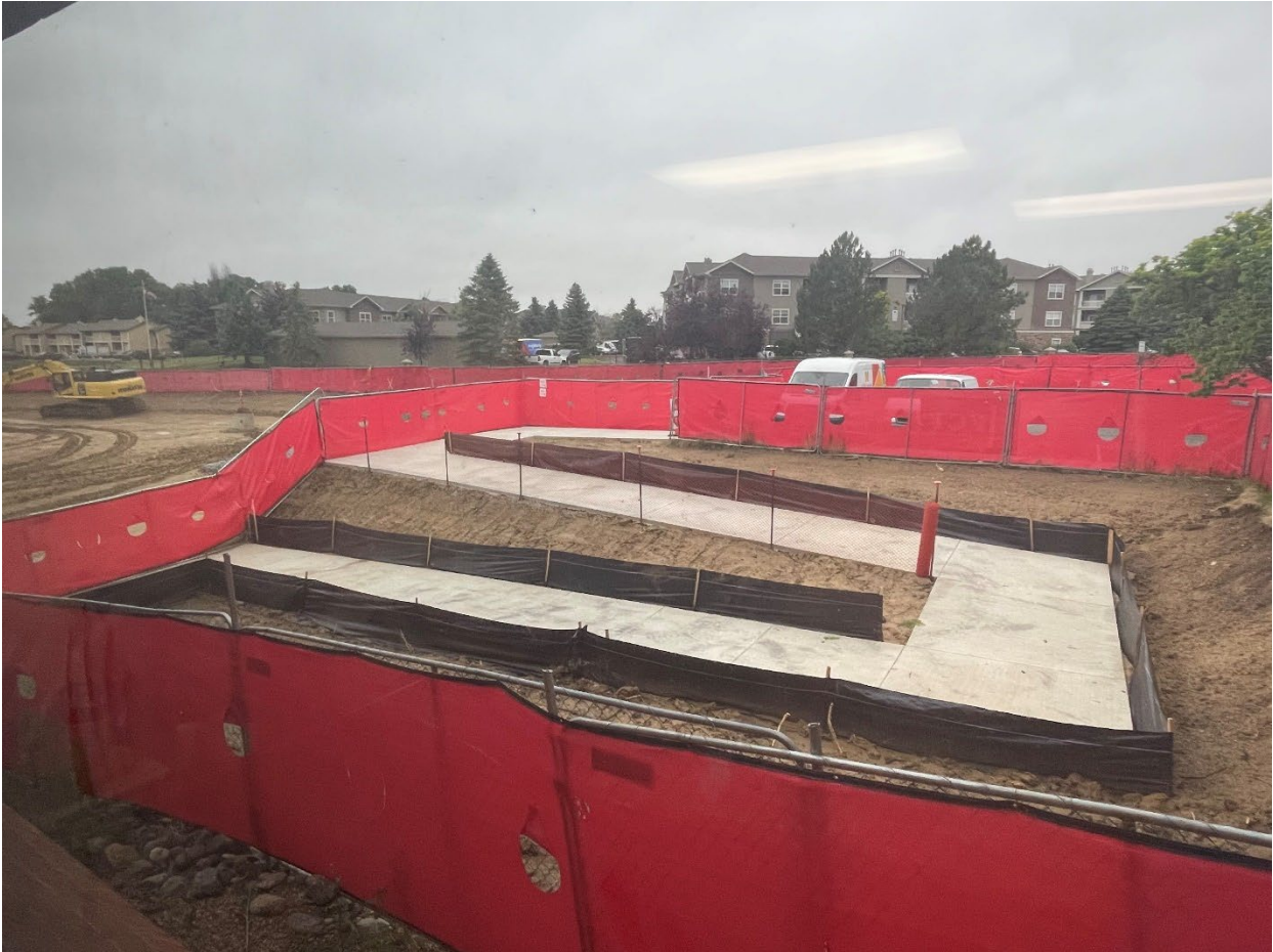
Photo 4 – Egress Sidewalk from East Lower-Level Door of Existing City Hall
