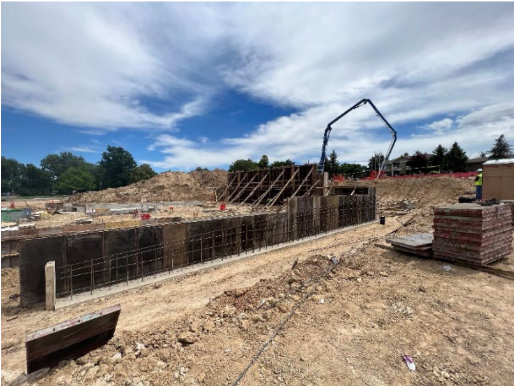
Photo 3 – Grade beam cast (facing SW)
