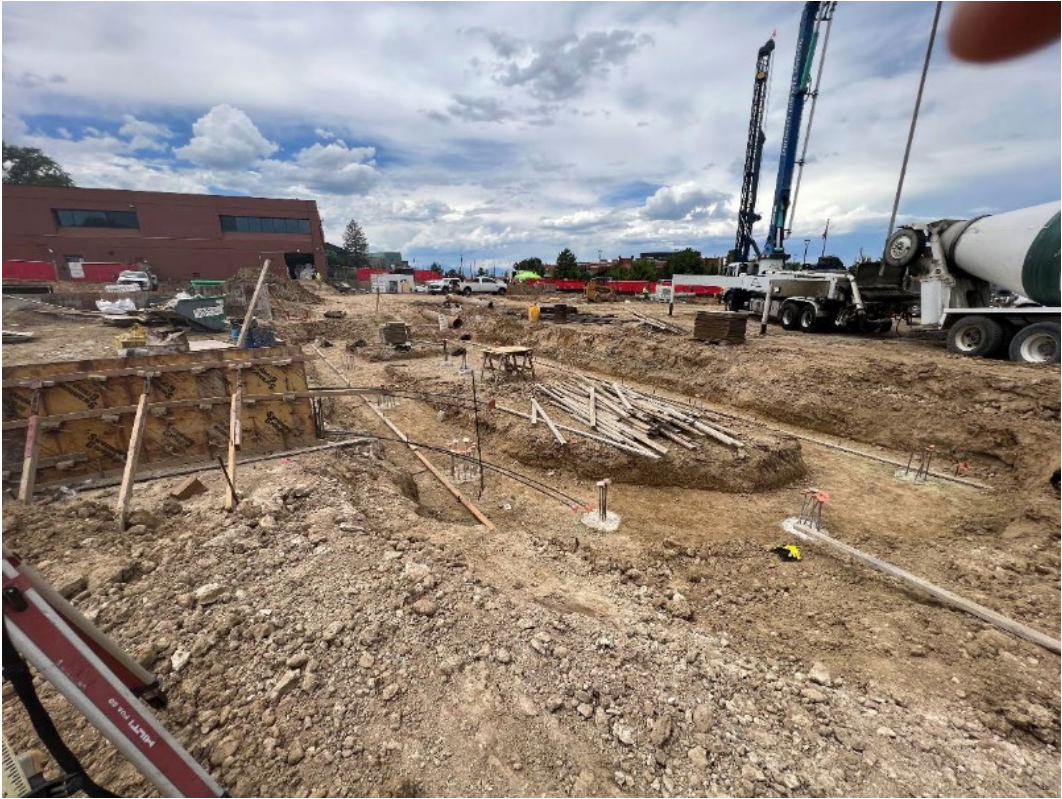
Photo 4 – Crawlspace excavation start
