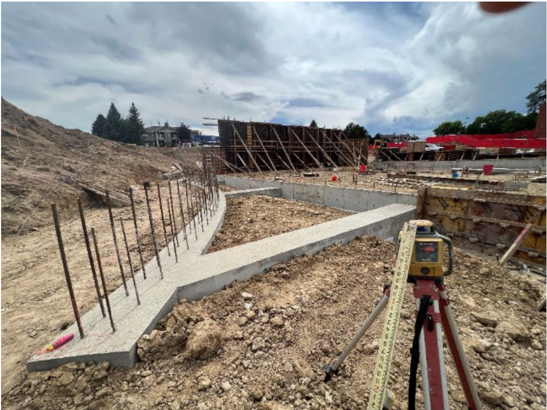
Photo 3 – Grade beam cast (facing SW)
