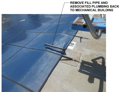
21 EXISTING POOL FILL LINE DETAIL VIEW T-100
