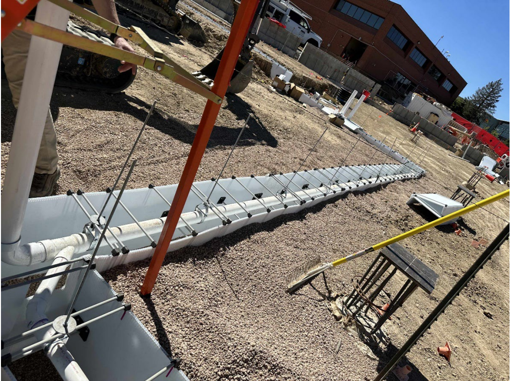
Photo 4 – Subgrade Suspended Utilities
