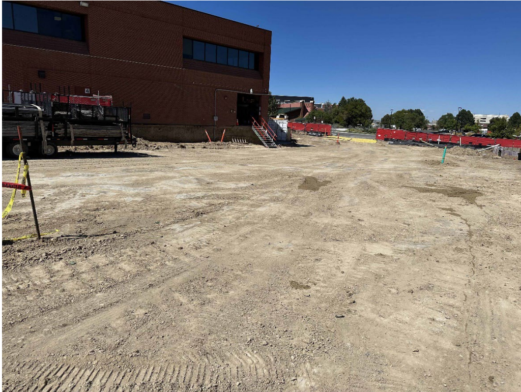
Photo 1 – Site Grading for Civic Way
