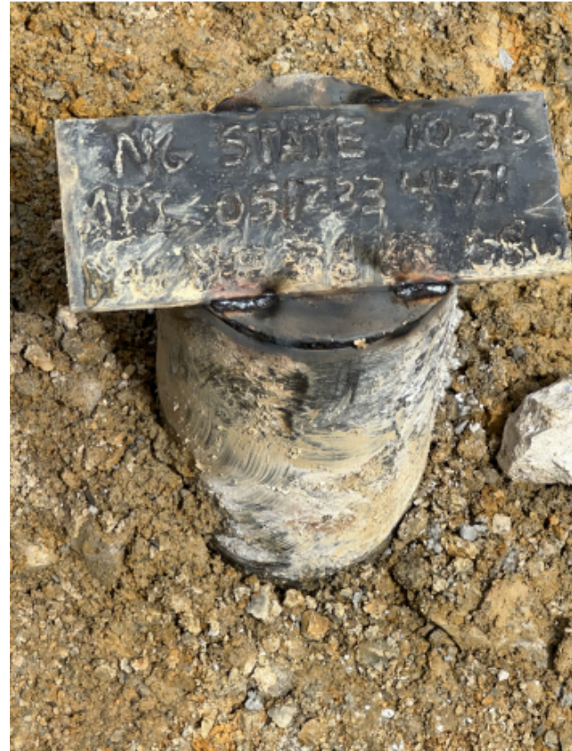
Cut & Cap Operations (cement verified at surface)
