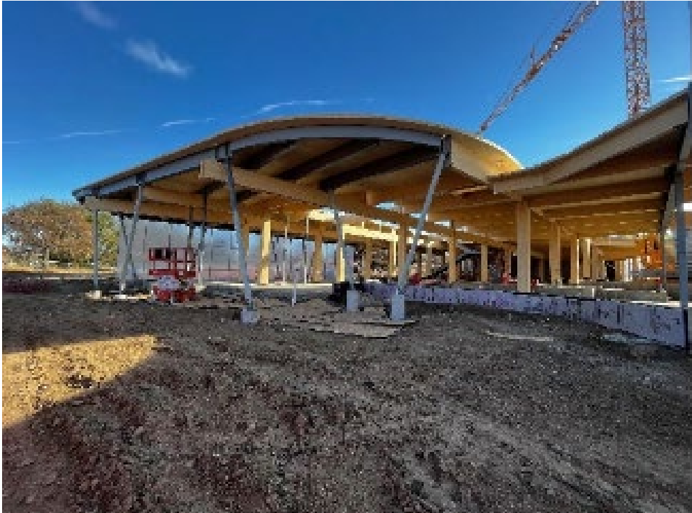
Photo 2 – Level 1 Steel and CLT (Facing SE)
