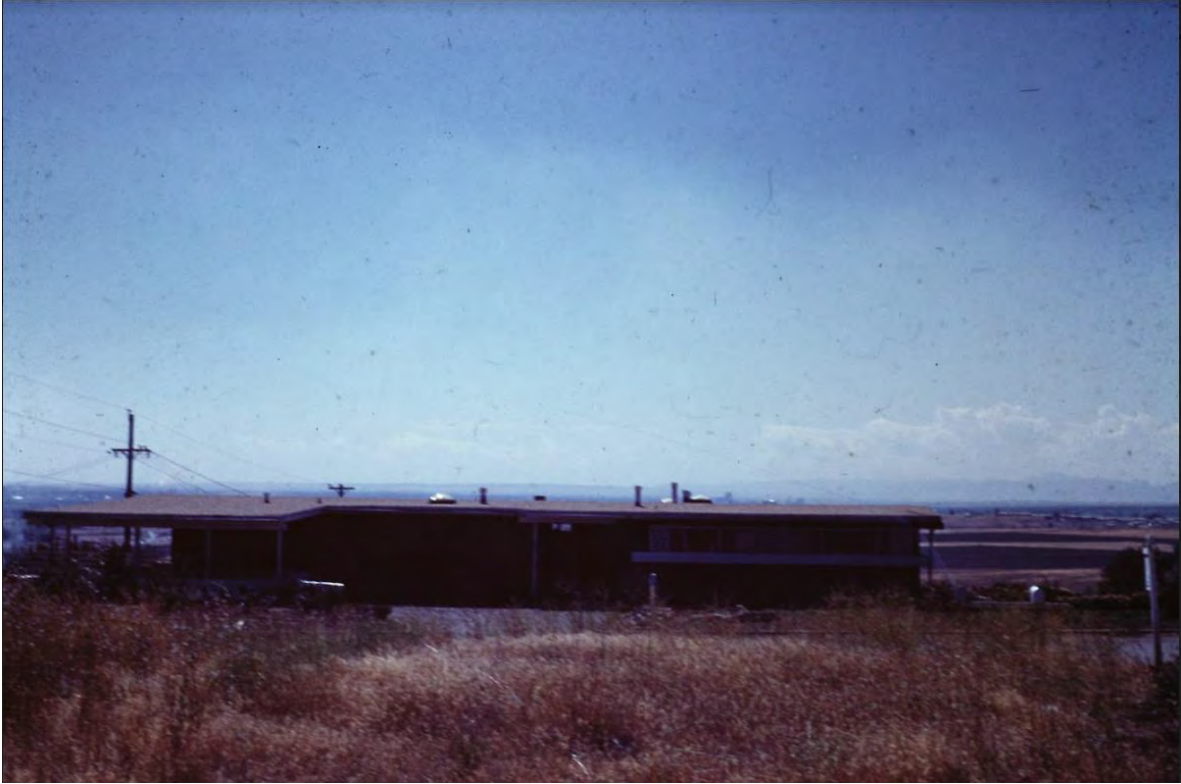
3 of 16: 880 W. 99 th Ave, exterior, date unknown.
