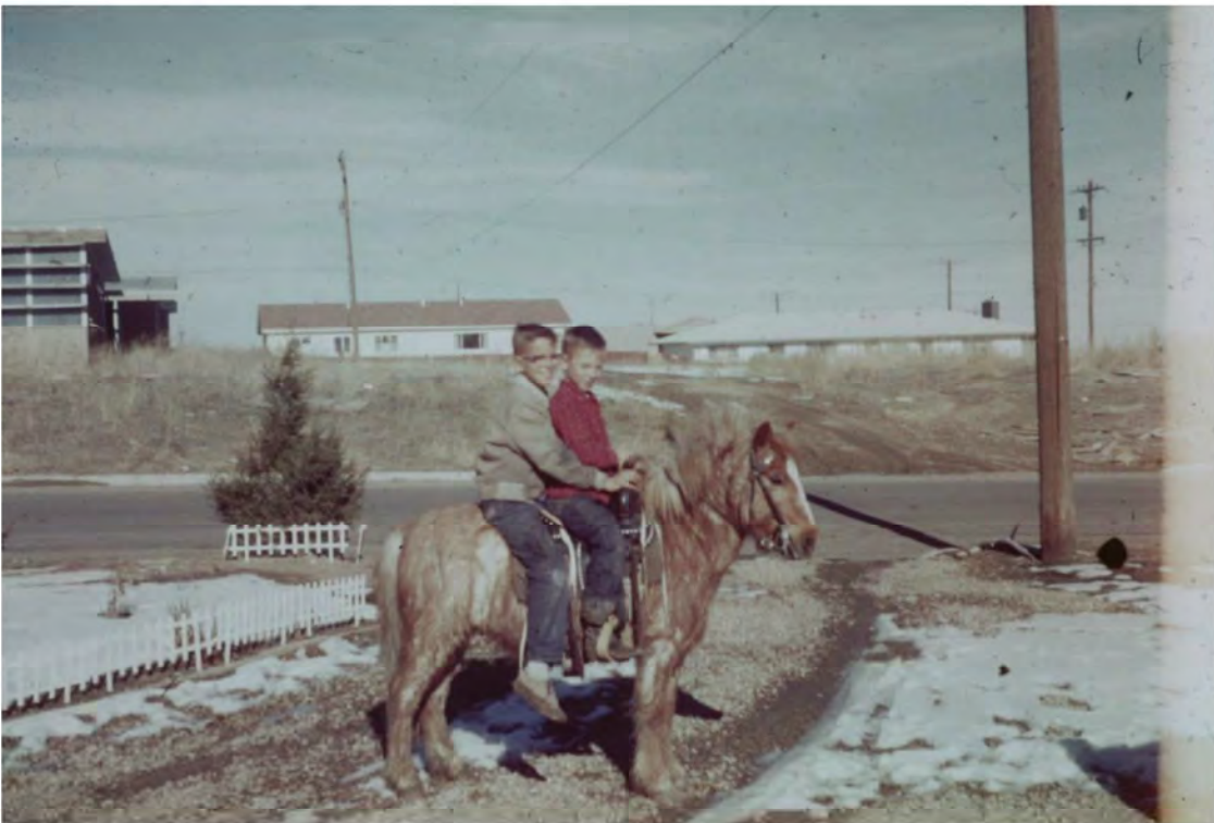
4 of 16: Residents of Deza Estates on horse, construction office locate at the northwest corner of Huron Street and W. 99 th Avenue in background, Photographer Donald Gravestain, date unknown.
