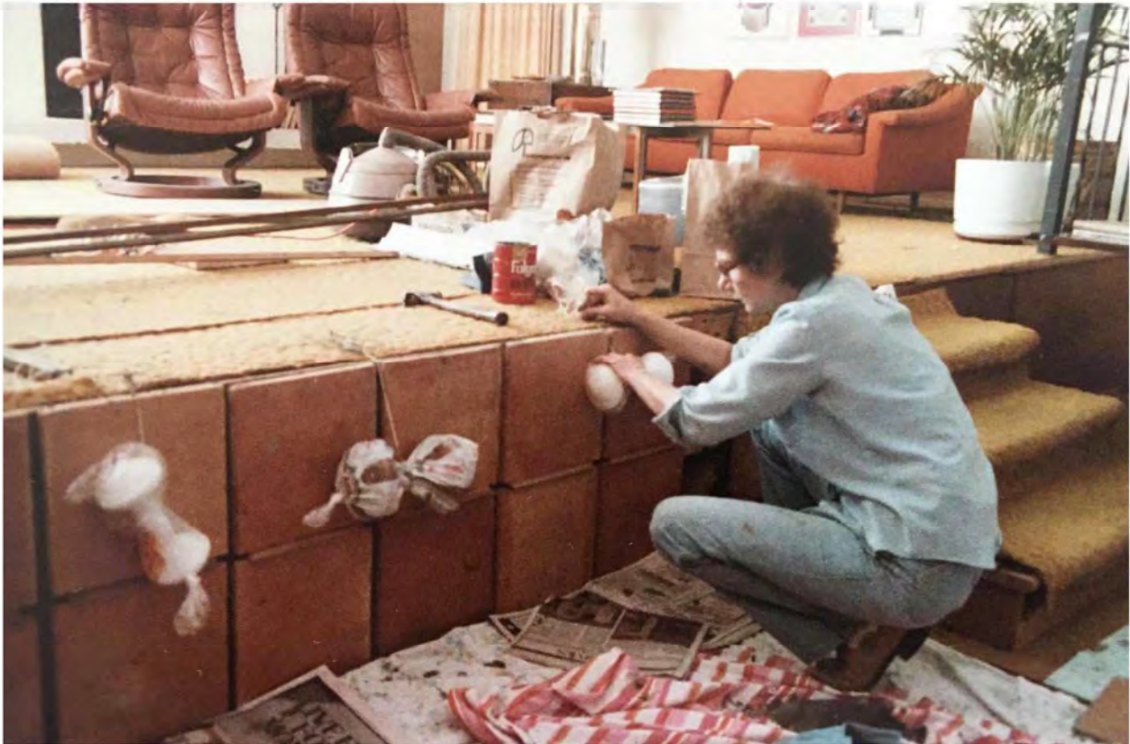
10 of 16: Patterson Home, Jo Patterson tiling living room platform, 9841 Rapp Lane, date unknown.
