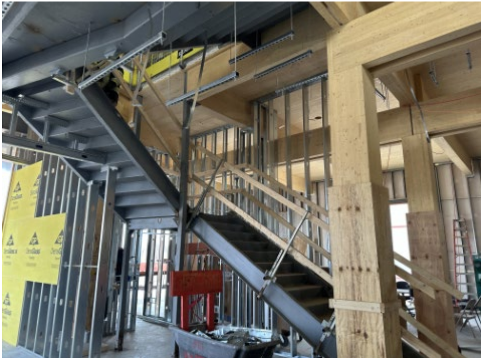
Photo 4 – Stairwell at Level 1 with MEP Supports and Framing
