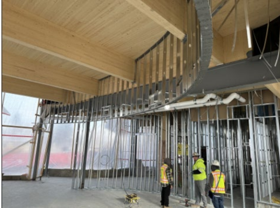
Photo 4 – Stairwell at Level 1 with MEP Supports and Framing
