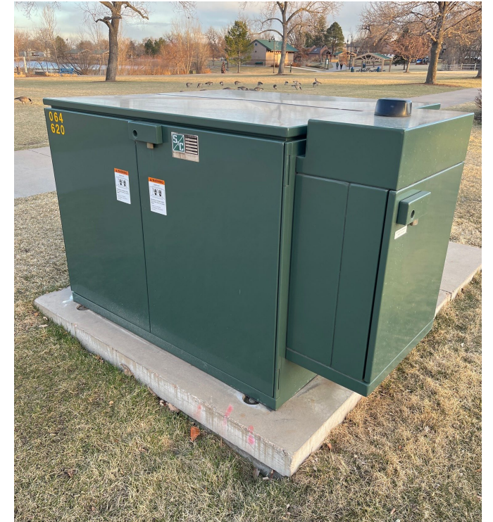
Wayfinding, Walkability and Vinyl Wraps Project
