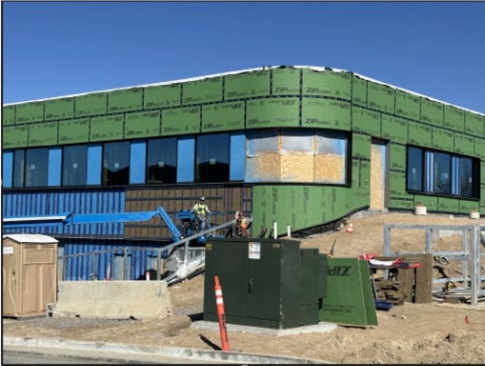
Photo 2 – Exterior Panel Underlayment (Facing ENE)
