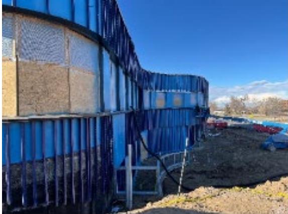
Photo 2 – Exterior Panel Underlayment (Facing ENE)
