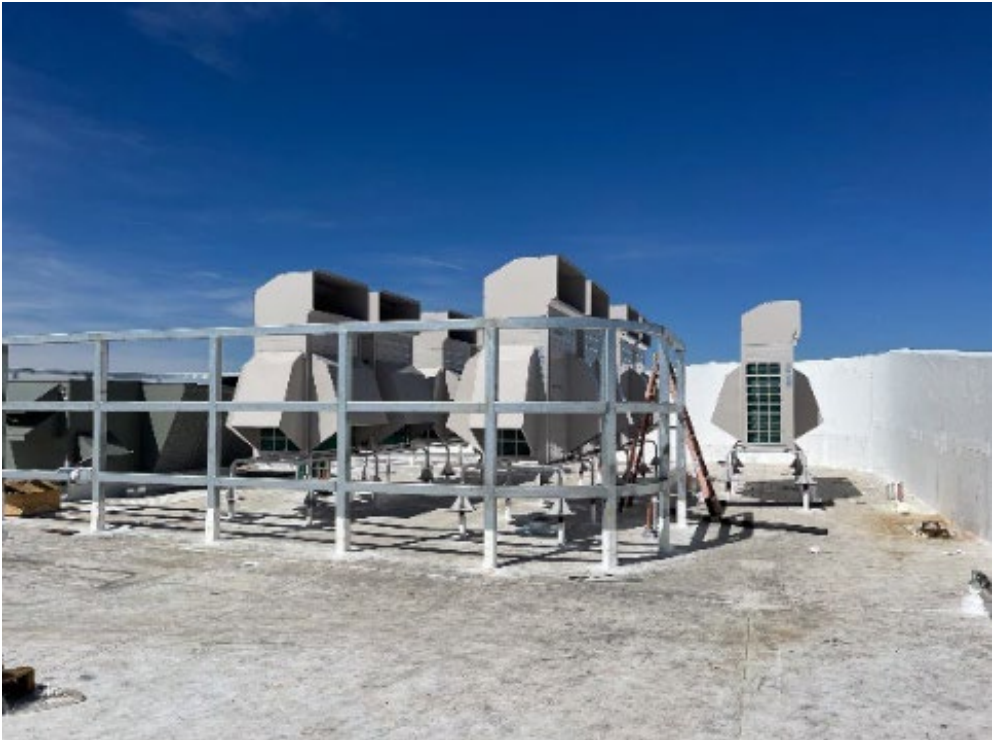
Photo 1 – Roof Mechanical and TPO Installation (Facing North)
