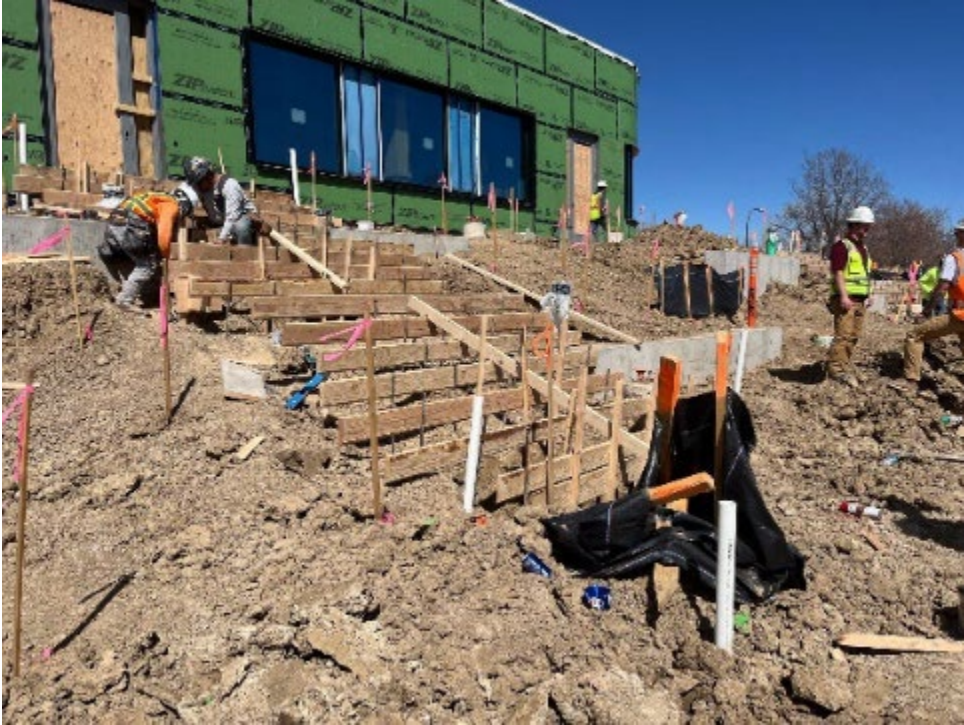
Photo 4 – South PV Canopy Prep and Stair Sidewalk Forming
