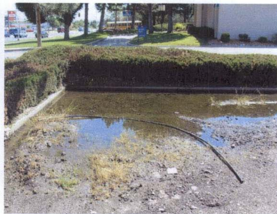
Makeshift Detention Pond
