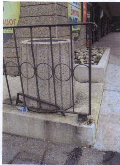
Broken Handrail
