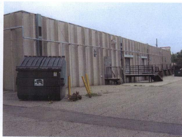
Alleyway of Inline Space
