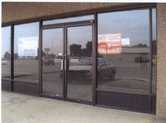
Vacant In-line Space
