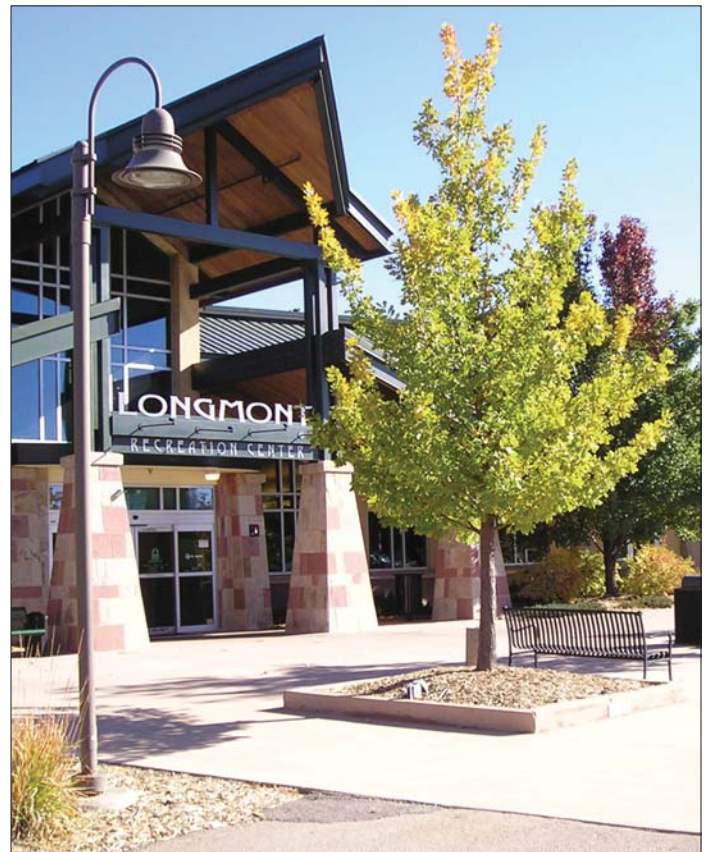
Entrance to the Longmont Recreation Center
