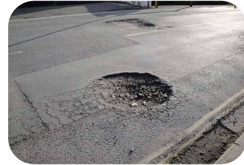
Potholes and Street Repair
