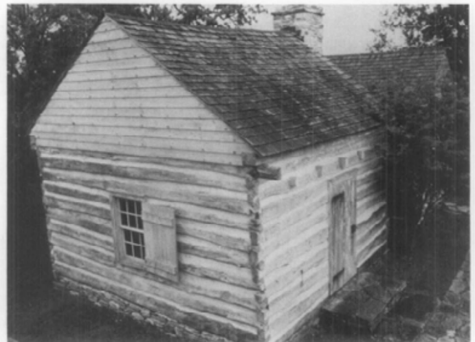
2. Handsplit and dressed shingles were also used on less elaborate buildings as seen in the restoration of the circa 1840 kitchen at the Winedale Inn, Texas. The uneven surfaces of the handsplit shingles were generally dressed or smoothed with a draw-knife to keep the rainwater from collecting in the wood grain and to ensure that the shingles lay flat on the sub-roof. Photo: Thomas Taylor.
