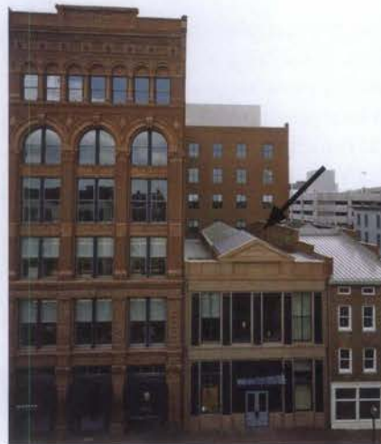
Figure 21. Both wings of this historic L-shaped building (top), which fronts on two city streets, adjoined vacant lots. A two-story addition was constructed on one lot (above, left) and a six-story addition was built on the other (above, right). Like the historic building, which has two different facades, the compatible new additions are also different and appear to be separate structures rather than part of the historic building.
