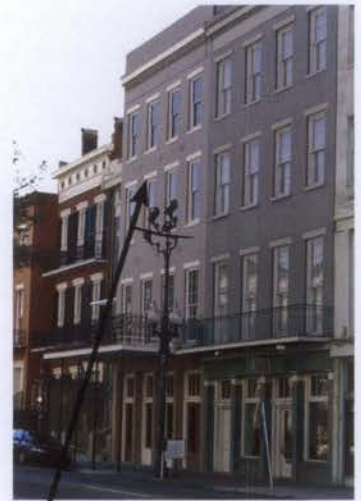
Figure 26. A rooftop addition would have negatively impacted the character of the primary facade (right) of this mid-19th century, four-story structure and the low-rise historic district. However, a third floor was successfully added on the two-story rear portion (below) of the same building with little impact to the building or the district because it blends in with the height of the adjacent building.
