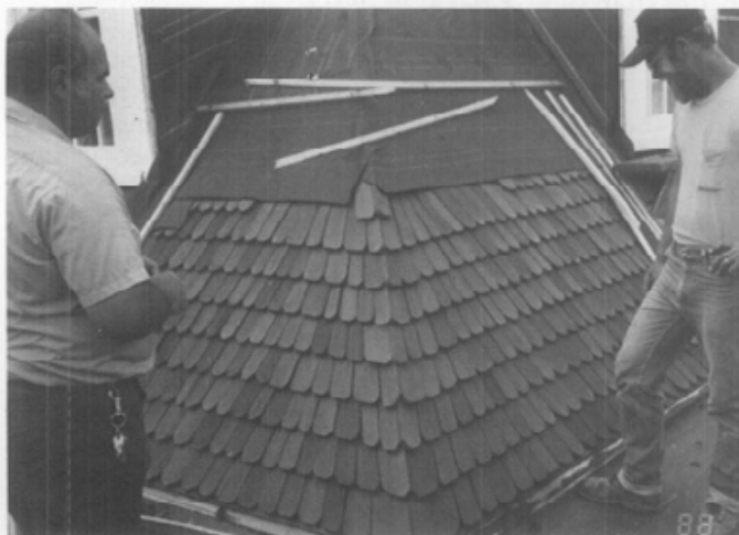
D. The fanned hips (seen here), swept valleys, and projecting ridge combs were installed as part of the re-roofing project. Special features, when documented, should be reproduced when re-shingling historic roofs.
