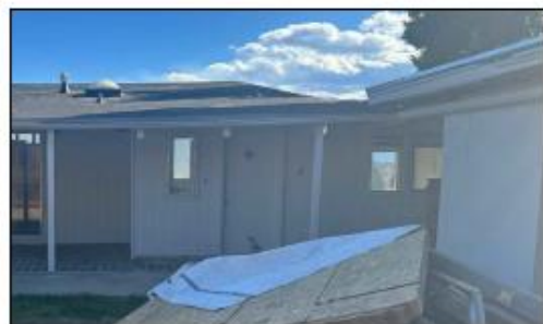
These doors and vestibule were not part of the original home.
