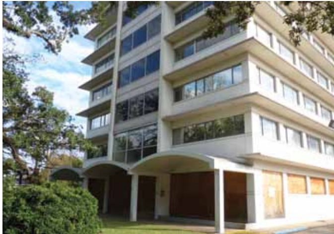
[4] Covered walkways and horizontal sun screens are distinctive and sustainable features in some mid-century modern office buildings.
