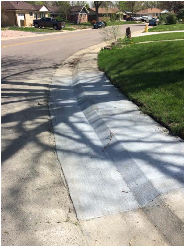
Concrete Repair Program
