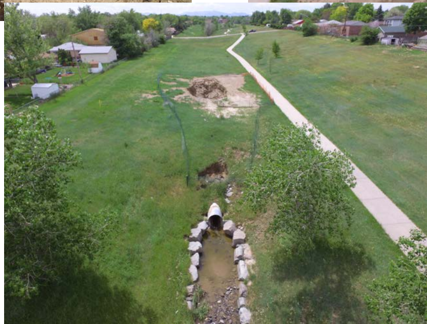
Grange Hall Creek Sinkhole / before conditions
