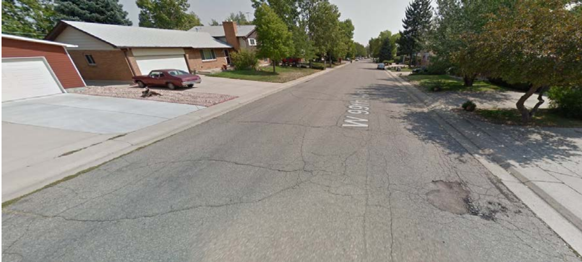
99th Avenue before reconstruction
