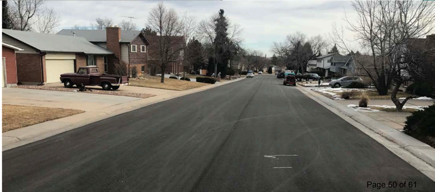
99th Avenue after reconstruction
