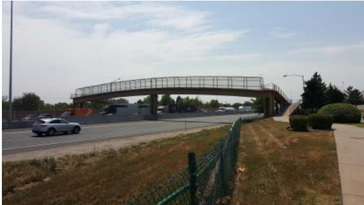
I-25 / Marketplace Pedestrian Bridge
