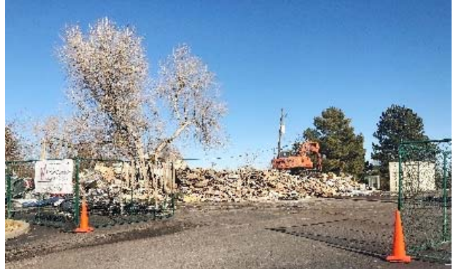
KFC demos building to start construction on its new modern restaurant at same location at 107 th & Washington St.
