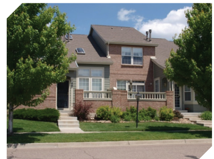
Residential development in Lowry development of Denver.
