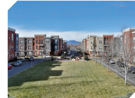
Residential development in Bradburn development in Westminster.
