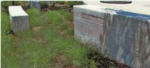
BOARDFORM FINISH CONCRETE SEATWALLS
