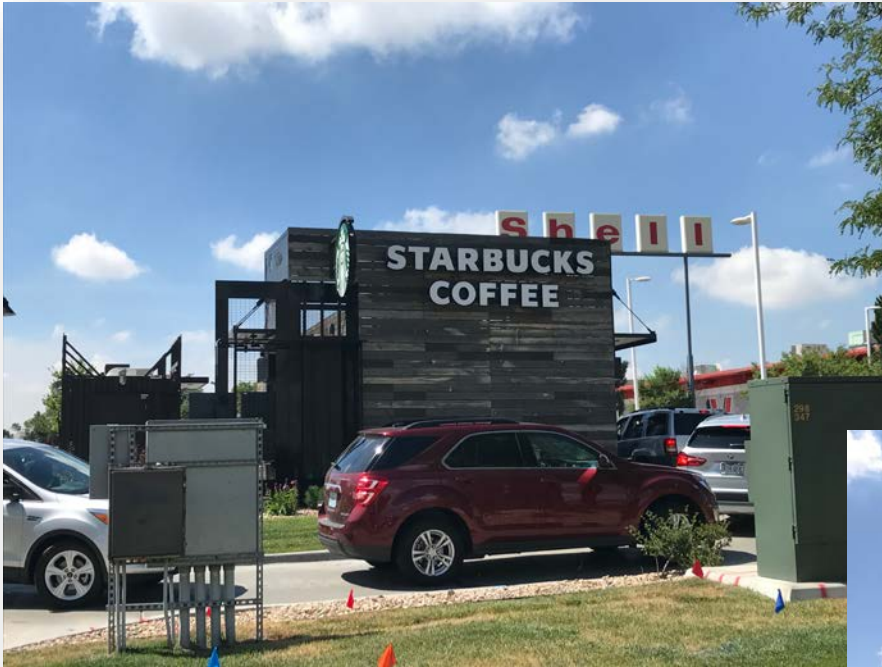
View of existing container store to be relocated.
