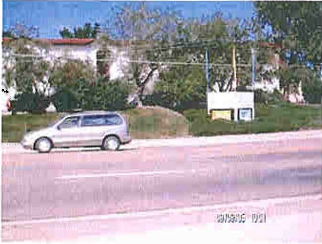
IMAG0042.JPG Storm Sewer Outfall Looking West
