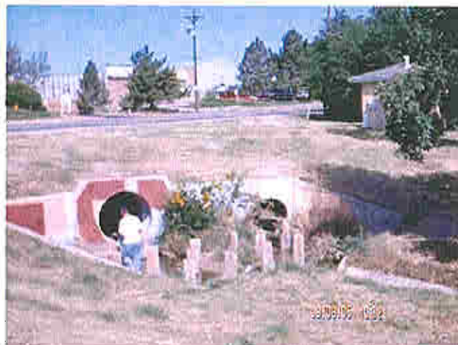
IMAG0045.JPG Storm Sewer Outfall
