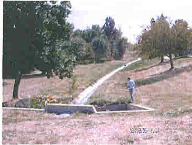
IMAG0043.JPG Storm Sewer Outfall Looking East
