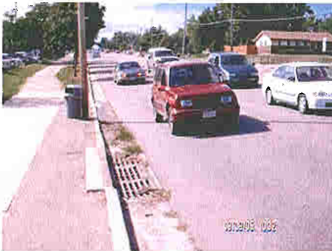
IMAG0044.JPG Inlets at Outfall
