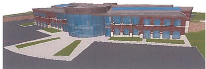
Subcontractor informational meeting to be held March 1 st at 9 a.m. on the new 45,000 s/f Justice Center facility.
