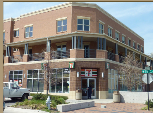
Example neighborhood-serving retail near station and at York St./112th Ave.
