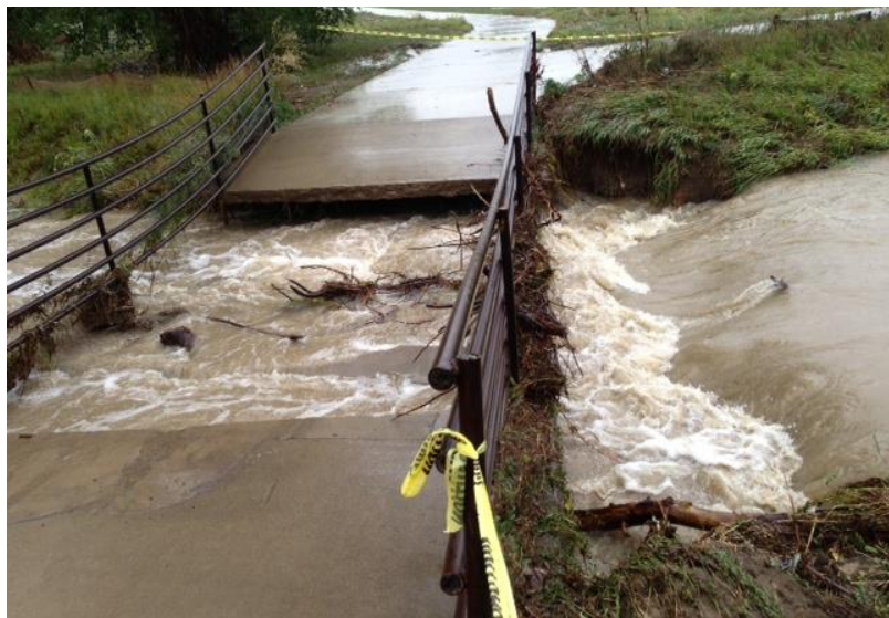
FIGURE 1. DAMAGES FROM 2013 FLOOD EVENT
