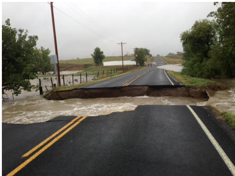
FIGURE 30. DAMAGES FROM 2013 FLOOD EVENT
