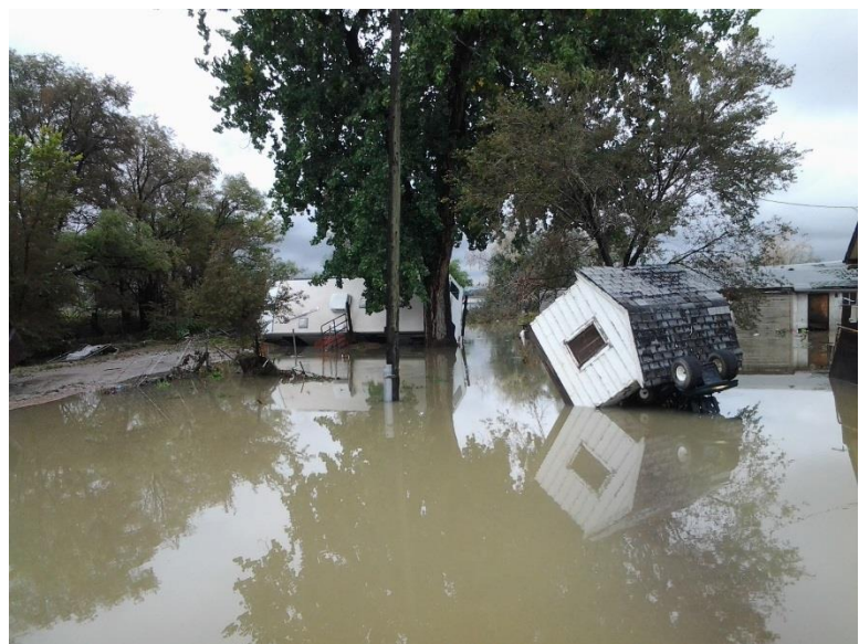
FIGURE 31. DAMAGES FROM 2013 FLOOD EVENT
