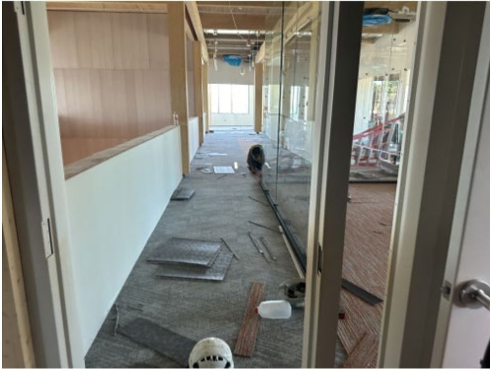
Photo 2,3 – Level 2 Carpeting Start
