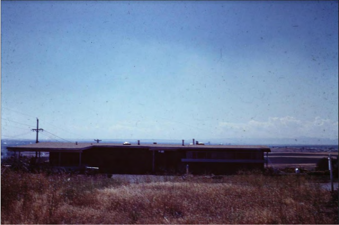
3 of 16: 880 W. 99 th Ave, exterior, date unknown.
