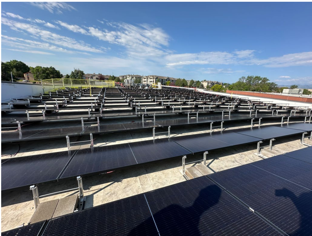
Photo 1 – Roof PV Array
