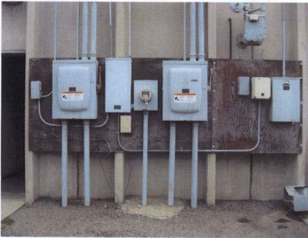
Electrical System Improperly Mounted to Rotting Plywood
