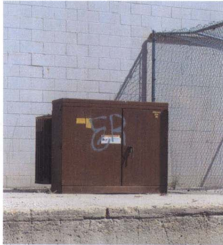
Graffiti on Utility Box
