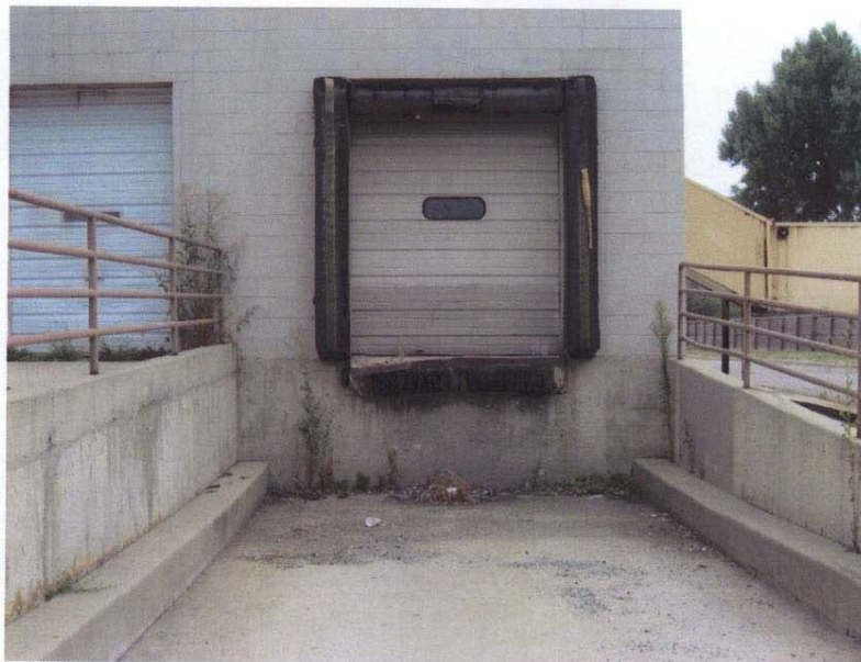
Deteriorating Loading Dock
