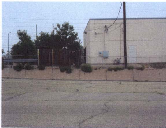
Slope of Parking Lot
