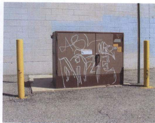
Graffiti on Utility Box
