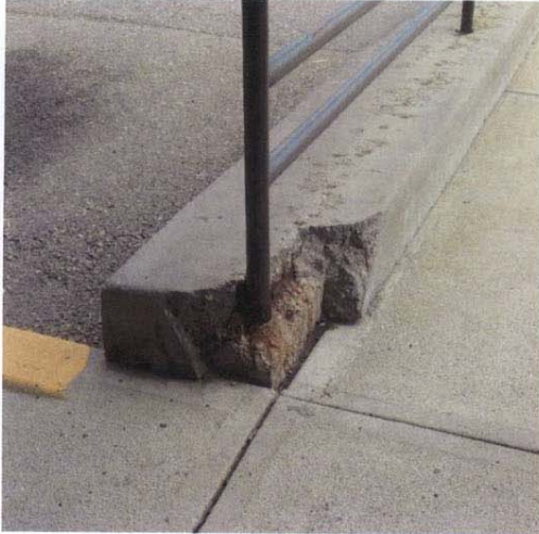
Broken Concrete
