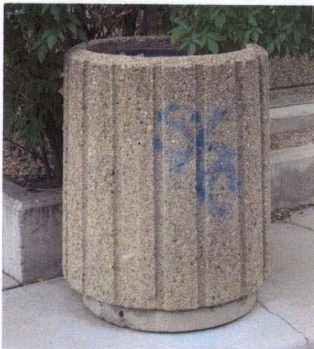
Graffiti on Trash Receptacle
