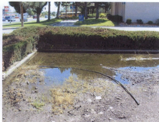
Makeshift Detention Pond
