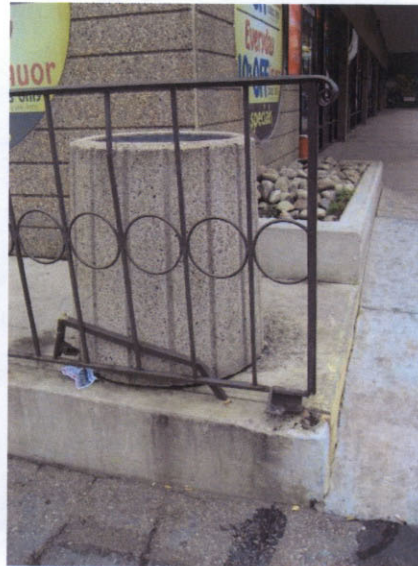
Broken Handrail
