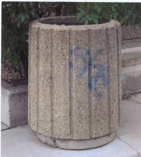
Graffiti on Trash Receptacle
