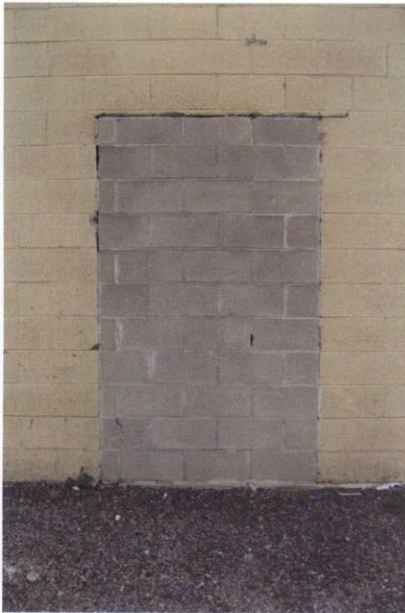
Doorway Permanently Sealed
