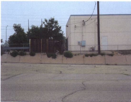
Slope of Parking Lot
