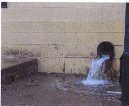
Roof Drain Emptying at Base of Building
